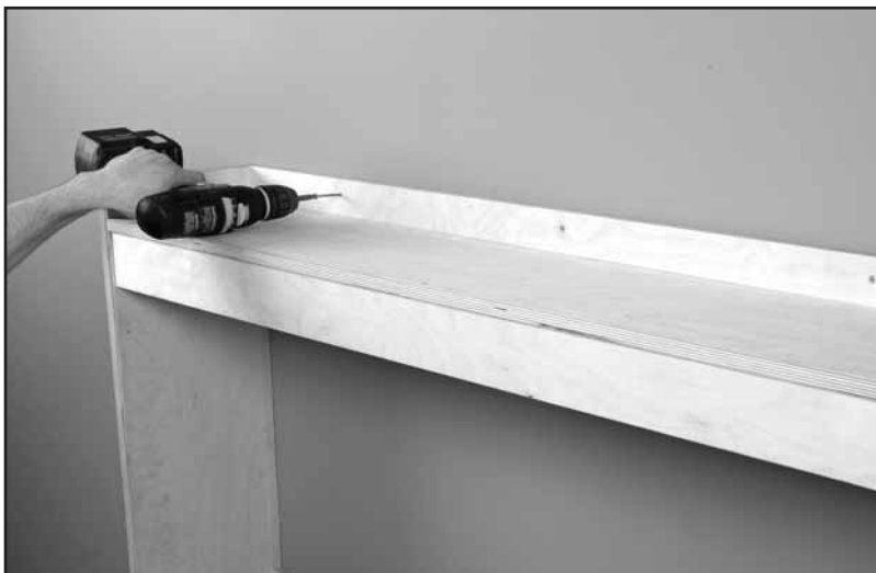
Fig. 7 - Use lag bolts for wall mounting (not included)
